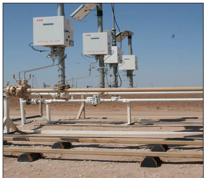
HBS-Base with 15/8" H-132 Pre-Galv. Steel Channel and Rollers
